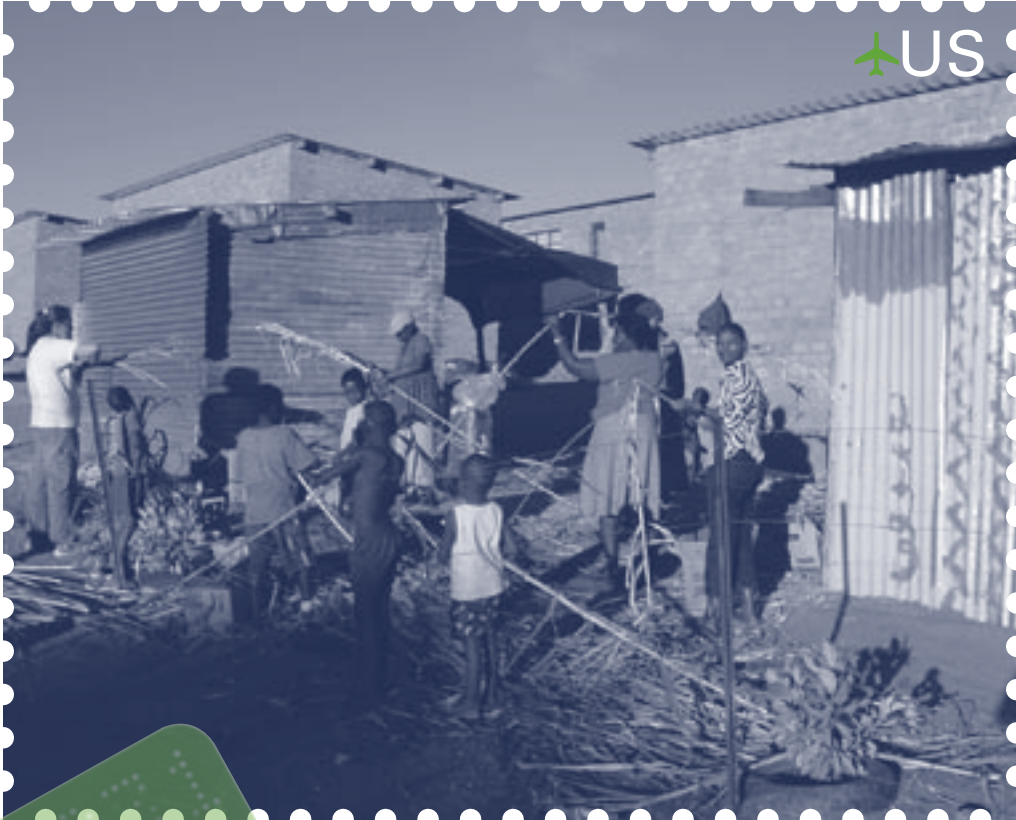
A Worcester Polytechnic Institute student working with residents of Goreangab, Windhoek, Namibia to improve the quality of shanty town housing
